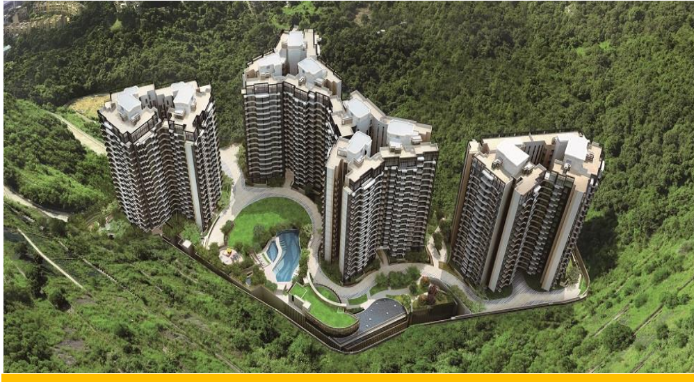
Dragons Range: Ten 30 storey towers & 970 units , waterproofed by Fosroc systems in all locations.
