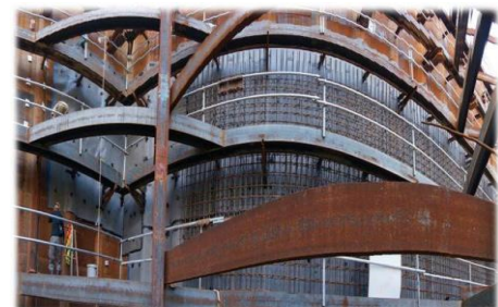
'Proofex Engage' applied on Basement (Pipe Pile Wall) & Floor Slab.
