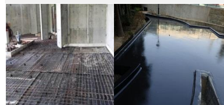
Left : 'Proofex Sheetdrain 100' in Basement internal & Planters. Right: 'Nitoproof 600PF' on roofs.
